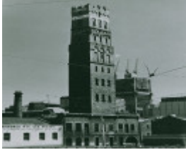
B0129 Coop's Shot Tower & Flanking Buildings Melbourne
