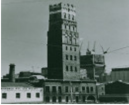
B0129 Coop's Shot Tower & Flanking Buildings Melbourne
