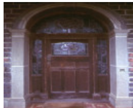
mt mitchell homestead & stables sunraysia hwy lexton front entrance nov84
