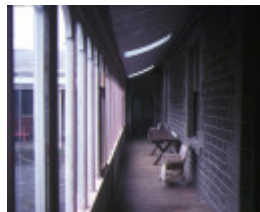
mt mitchell homestead & stables sunraysia hwy lexton verandah jul83
