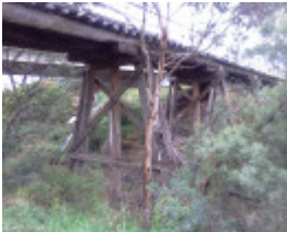
B3737 Trestle Bridge Keilor
