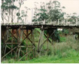
B3737 Trestle Bridge Keilor
