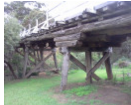
B3737 Trestle Bridge Keilor
