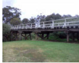
B3737 Trestle Bridge Keilor 2012
