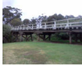
B3737 Trestle Bridge Keilor 2012
