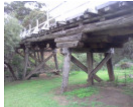
B3737 Trestle Bridge Keilor
