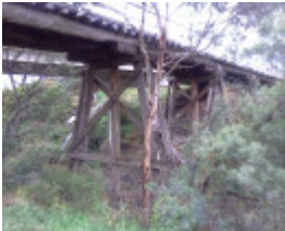
B3737 Trestle Bridge Keilor
