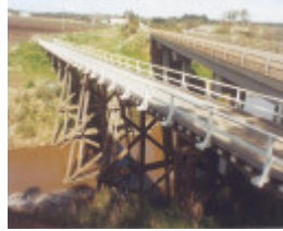
B3737 Trestle Bridge Keilor
