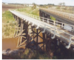
B3737 Trestle Bridge Keilor
