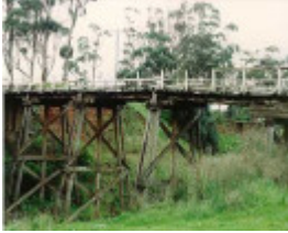
B3737 Trestle Bridge Keilor
