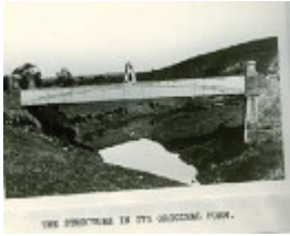
B1836 Iron Bridge
