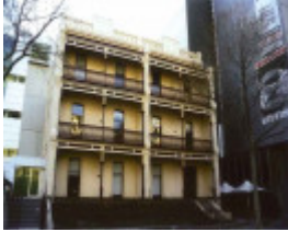
B6622 Former Lonsdale Private Hospital
