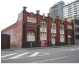
B6623 Reidys Building
