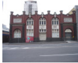
B6623 Reidys Building
