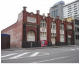
B6623 Reidys Building
