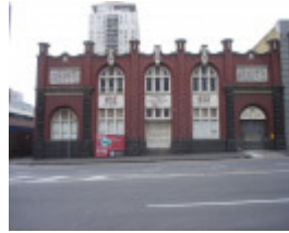
B6623 Reidys Building
