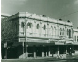
B3518 Tilley's Building
