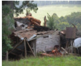
B3239 Storm Damage March 2012
