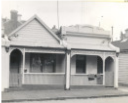
B0750 Pair of Timber Houses
