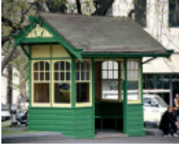
B4747 Tram Shelter
