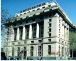
B4119 Fmr Port Authority Building
