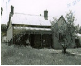
B3598 65 Frawley Road
