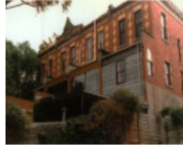
B6892 Rear Facade
