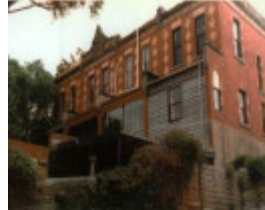
B6892 Rear Facade
