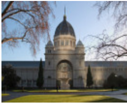
B0842 REB and Museum Victoria Verandah
