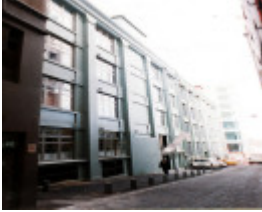
B7005 Warehouses Oliver Lane
