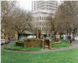
B6791 Underground Public Conveniences
