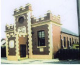
B6828 Former Salvation Army Barracks
