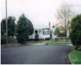
B6526 Railway Workers Cottages
