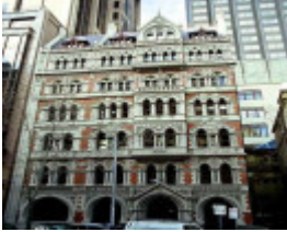
B3574 Safe Deposit Building
