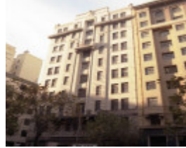
B6190 Vaughan Building
