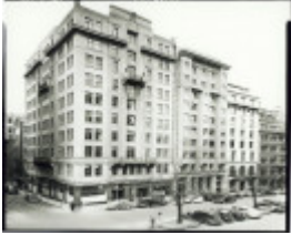
B6190 Vaughan Building
