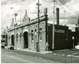
B5342 Cable Tram Engine House & Car Shed
