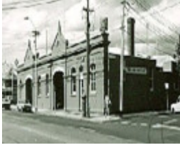
B5342 Cable Tram Engine House & Car Shed
