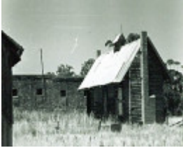
B3753 Police Stud Buildings
