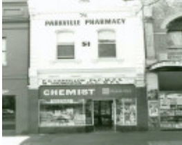
B4721 Frmr Parkville Pharmacy Facade
