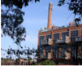
B2321 Yarra Falls Chimney
