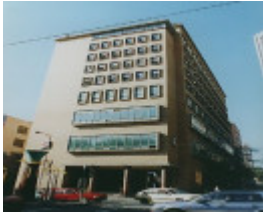
B6992 Former Telephone Exchange Post Office
