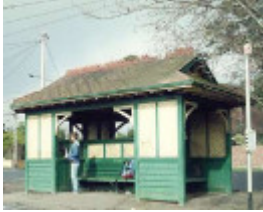
B7040 Tram Shelter
