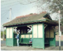
B7040 Tram Shelter
