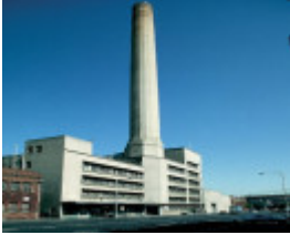
B6614 Lonsdale Street Power Station.
