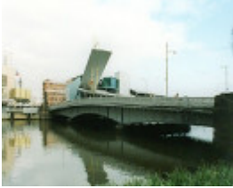
B6799 Spencer Street Bridge
