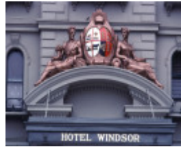
B0423 Hotel Windsor Entrance
