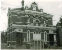
B5653 Post Office Elsternwick
