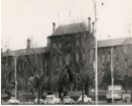
B1255 Victoria Barracks A Block
