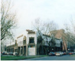
B4870 Former Car Showroom
