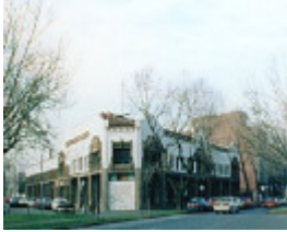
B4870 Former Car Showroom
