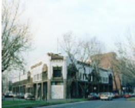
B4870 Former Car Showroom
