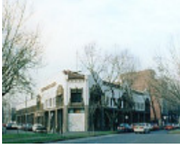
B4870 Former Car Showroom
