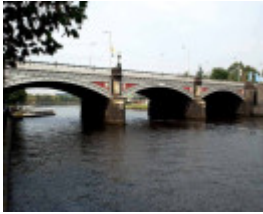
B2238 Princes Bridge
