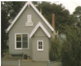
little hampton primary school no 1700 side view
