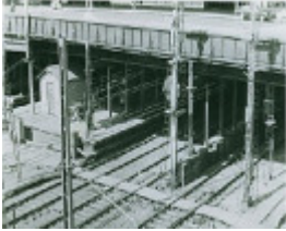
B3120 Swanston St Bridge Over Rail Lines
