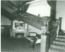
B5468 Dacre Staircase
