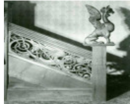
B5468 Dacre Staircase Detail
