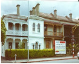
B5067 66-74 Toorak Road West
