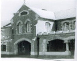
B2715 Clarke Building Trinity College Parkville
