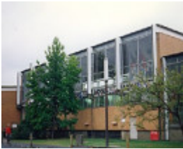
B6318 Beaurepaire Building
