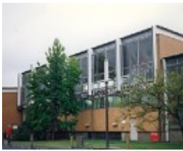
B6318 Beaurepaire Building
