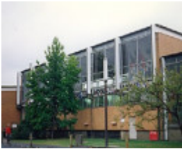
B6318 Beaurepaire Building
