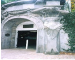
B6479 Underground Carpark
