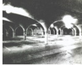
B6479 Underground Carpark
