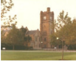
B6489 Old Arts Building
