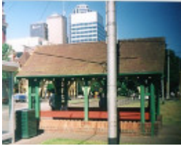
B7050 Tram Shelter
