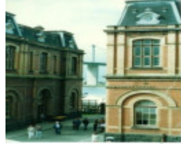
B3704 Spotswood Pumping Station
