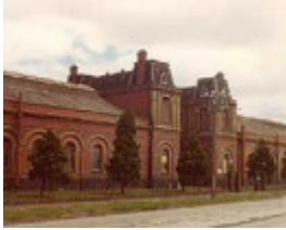
B3704 Pumping Station
