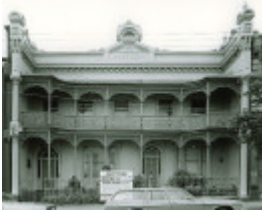
B2916 Victoria Crescent 442 Victoria St Nth Melbourne
