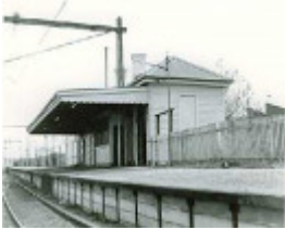
B4023 Williamstown Pier Station
