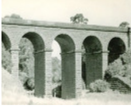
B1787 Railway Viaduct, Sunbury
