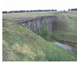
B3033 Bolinda Railway Viaduct 2011
