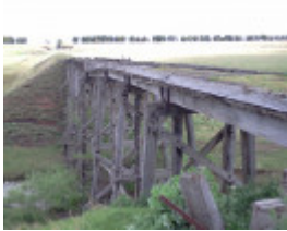
B3033 Bolinda Railway Viaduct 2011
