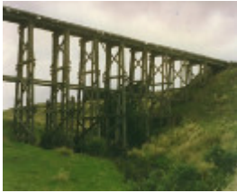
B3033 Bolinda Creek Railway Viaduct
