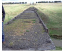
B3033 Bolinda Railway Viaduct deck 2011
