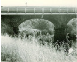
B3039 Bluestone Road Bridge
