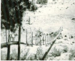
B2230 Catenary Bridge
