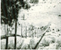
B2230 Catenary Bridge
