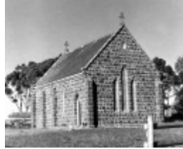
B2378 St Mary's C of E at New Site
